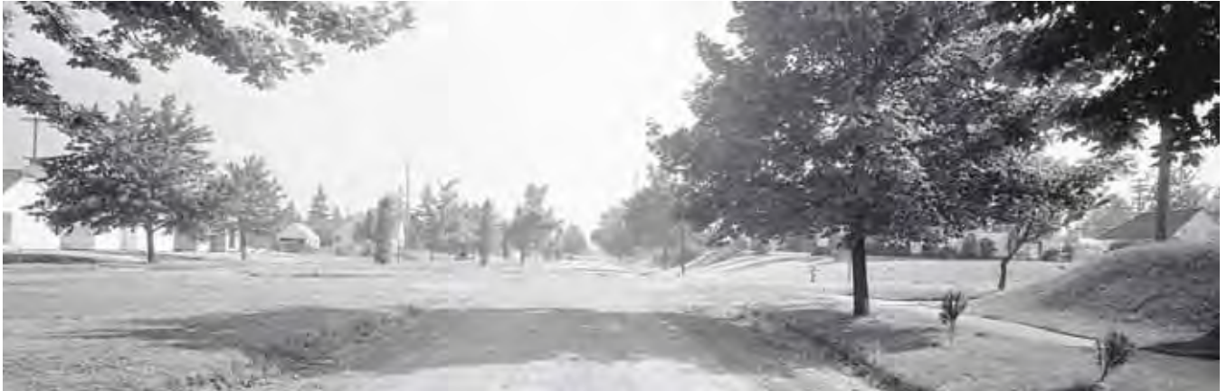
1941Aug18 - N 21st Street & Union Avenue, view south district on left, Tacoma Public Utilities Collection
