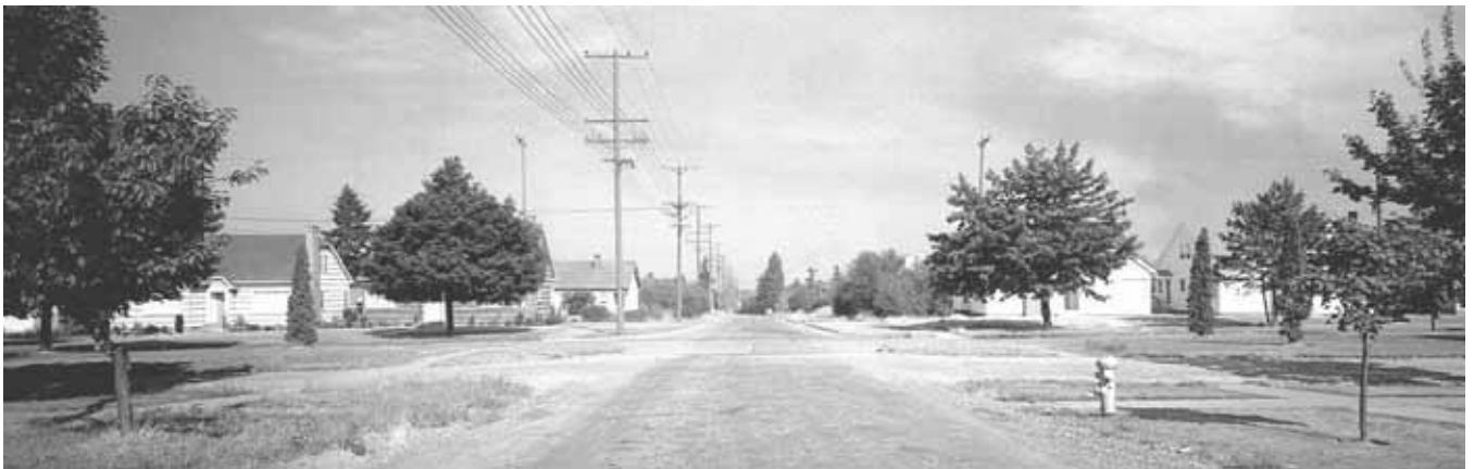
1941Aug18 - N. 21 st Street & Union Avenue, view east district on right, Tacoma Public Utilities Collection
